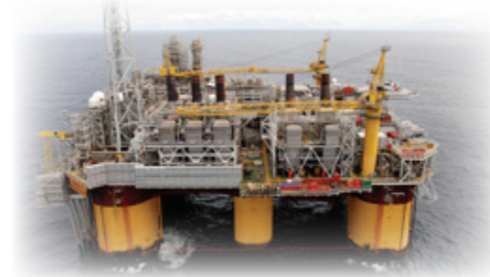
Planta Off-Shore (Noruega) Off-Shore plant (Norway)
